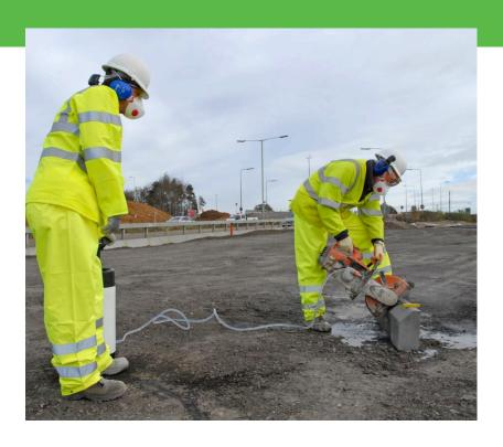
Water suppression systems fitted to tools usually involve spraying water directly onto the material. The water spray is supplied via mains water supply or a pressurised water bottle. There needs to be an adequate supply of water so make sure you have this before you start. Pouring from a container before you start will not be sufficient.
