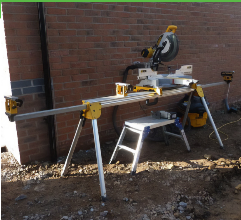
Picture illustrates chop saw fitted with dust extraction.
